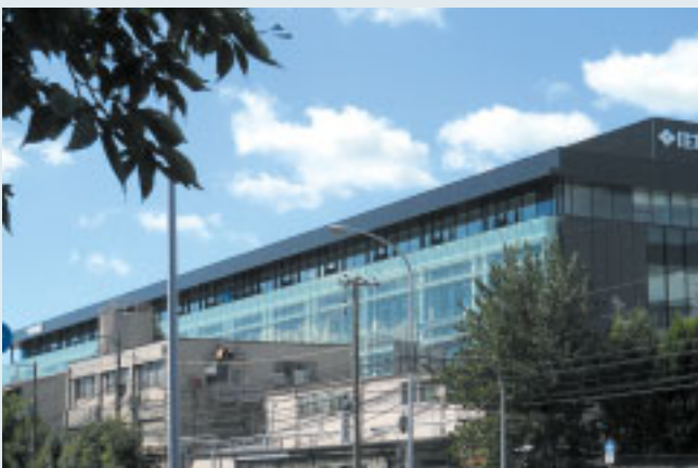
ビル外壁パネル (タナカ-P4) Exterior wall panels of buildings (Tanaka-P4)
