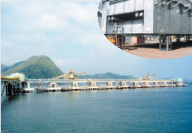
積出し棧橋 桁 Shipping pier girders
