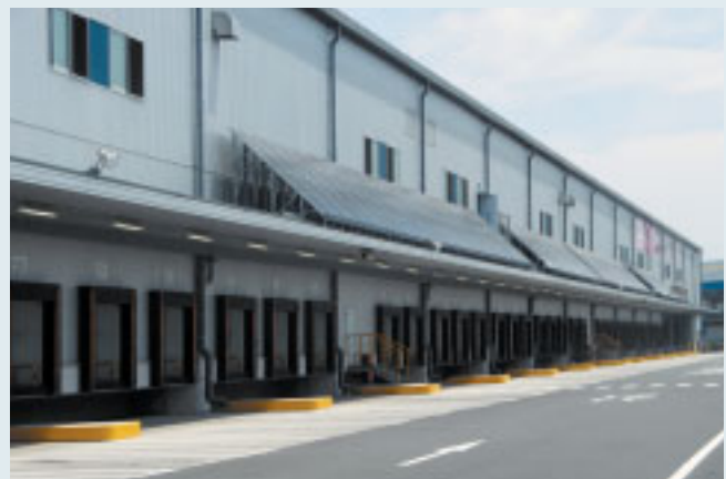
物流倉庫 鉄骨 Iron frames for distribution warehouses
