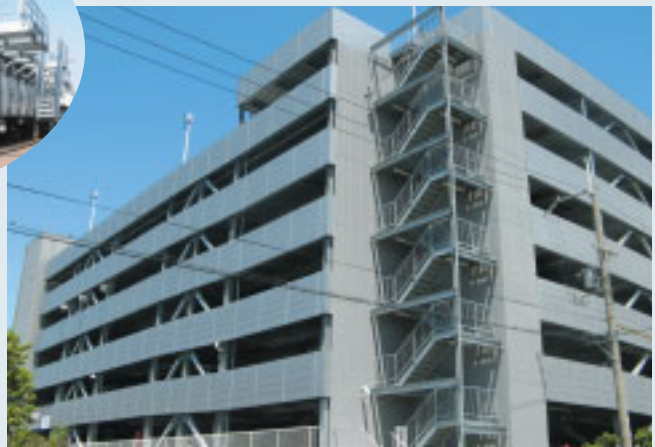
自走式立体駐車場 鉄骨 Iron frames for self-propelled multilevel car parking towers
